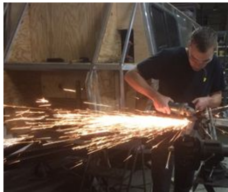
Figure A.5. Hand Grinding of The Sheets.
